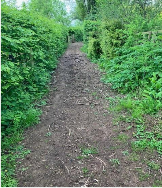
Photo 15. HU 10.2-3 (April 2025) Improved drainage.
