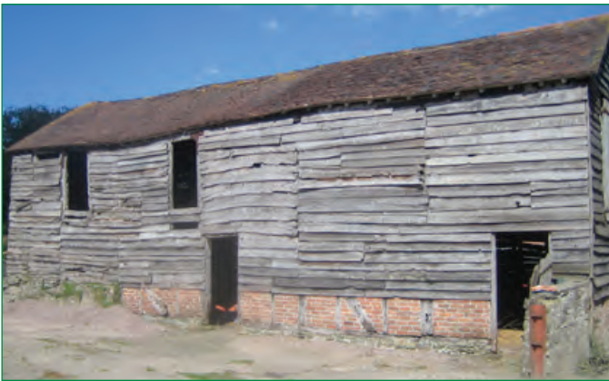
An example of storeyed cattle housing in weatherboarded timber frame. The Plateau includes some very rare examples of 18th century and earlier cattle housing, as found elsewhere along the Welsh borders.
