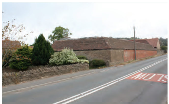
A large U-plan range, with cattle housing in the foreground and a large barn range to the rear.
