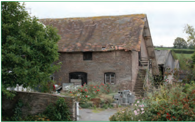
A first-floor granary, marked by its external steps, above a ground floor cider house marked by its wide doorway for taking barrels.
