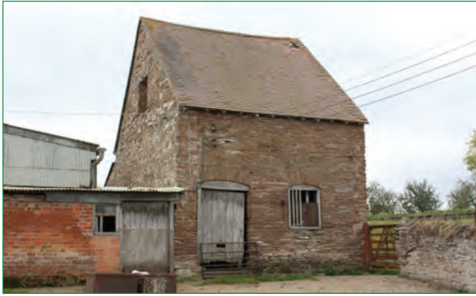
A first-floor granary, marked by its external steps, above a ground floor cider house marked by its wide doorway for taking barrels.
