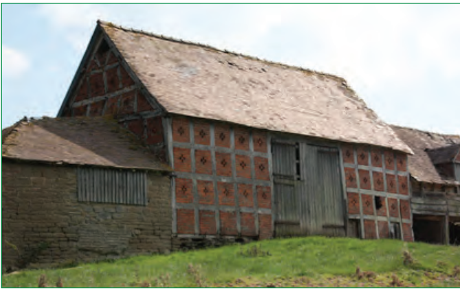
Barns were typically of 5 bays. This example displays the square panel timber framing found along the Welsh borders.
