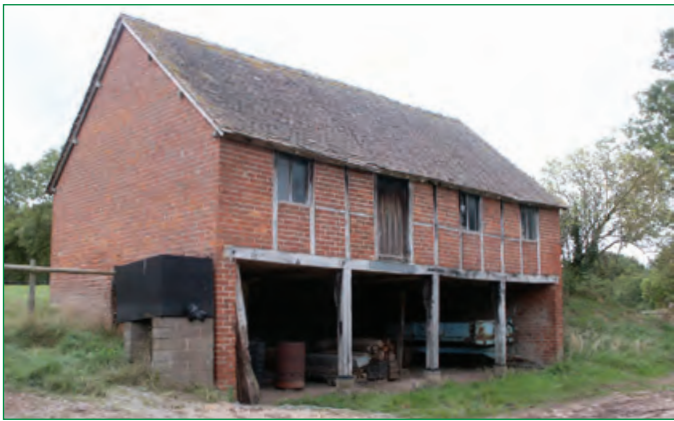
A large granary located above a 4 bay cartshed indicative of the importance of arable on this farm.
