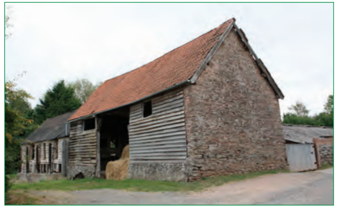
Barns were often built with stone gable ends and weatherboarded timber to the storage bays.
